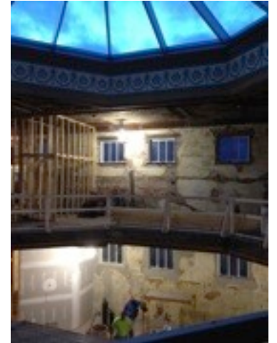
Atrium Skylight at dusk Waiting to install the railings
