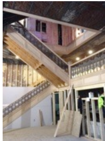
Atrium Grand Staircase & balcony Staircase to 3rd floor from atrium
